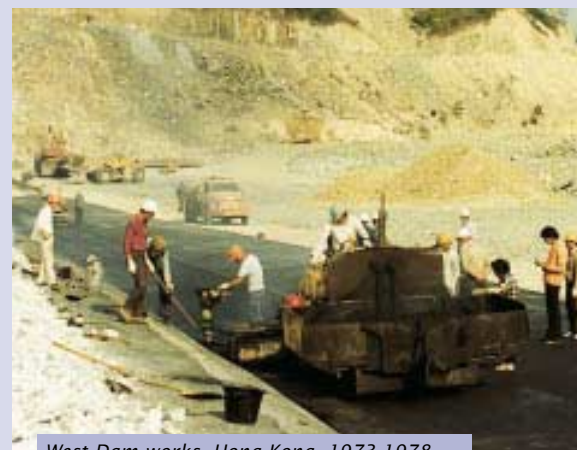
West Dam works, Hong Kong, 1973-1978
